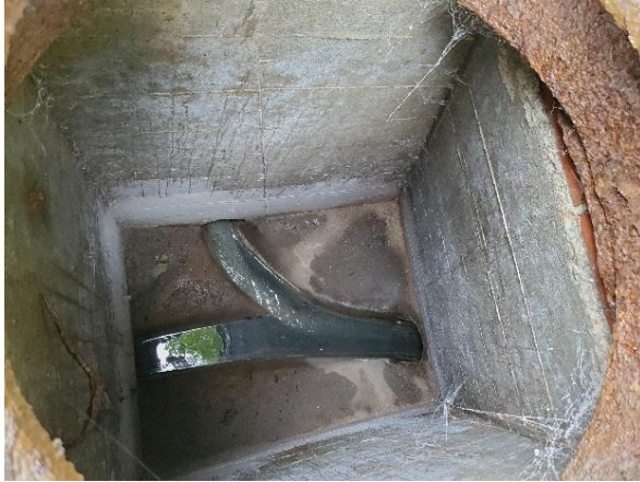
Figures 4. Typical manhole ready for reuse
