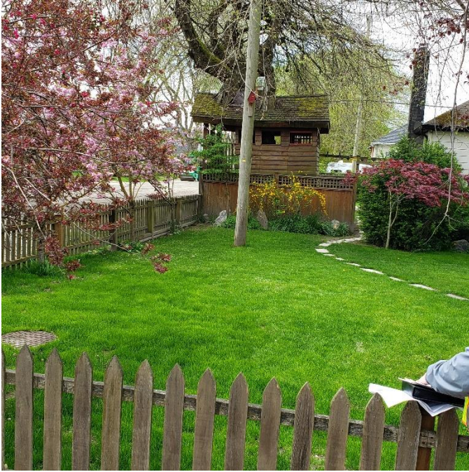
Figure 2. Shows the alignment of sanitary sewer between the manhole and middle of treehouse
